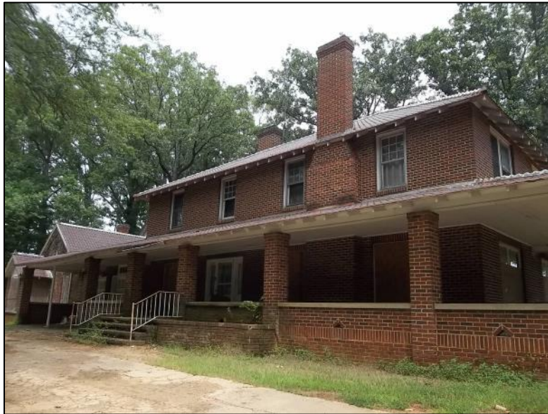
Photo 40: West (Primary) Elevation of the Dr. H.W. Barrier House.
