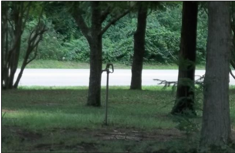
Photo 80: Pump, Looking Northwest.
