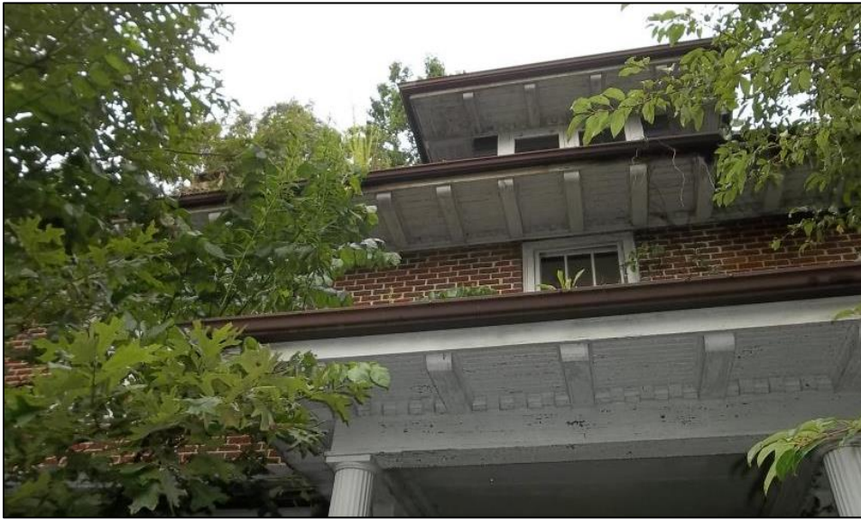
Photo 3: Detail of Eaves on the East Elevation.
