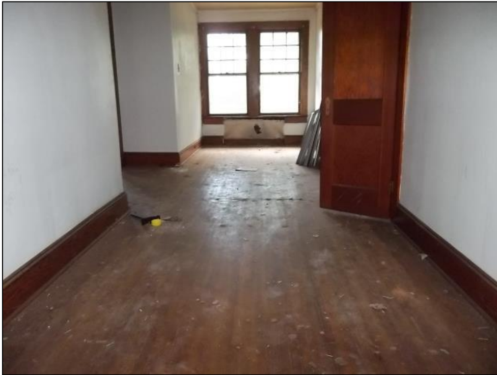
Photo 66: Hallway on the Second Floor, Looking South.
