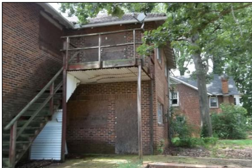
Photo 47: South Elevation of the Two-Story Addition.
