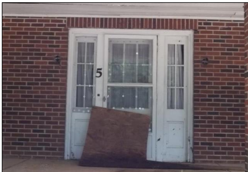
Photo 43: Primary Entrance on the West Elevation.
