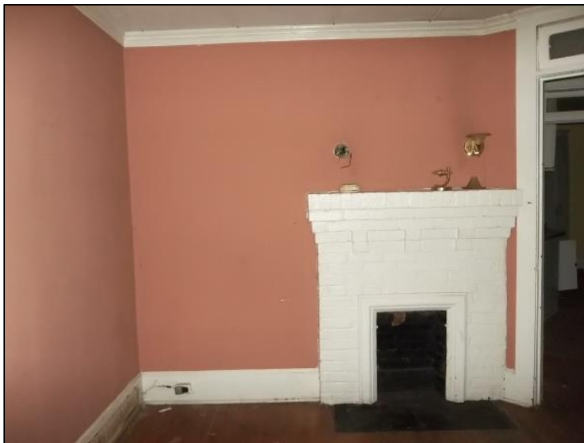
Photo 74: Northwestern Office and Fireplace Detail, Looking East.
