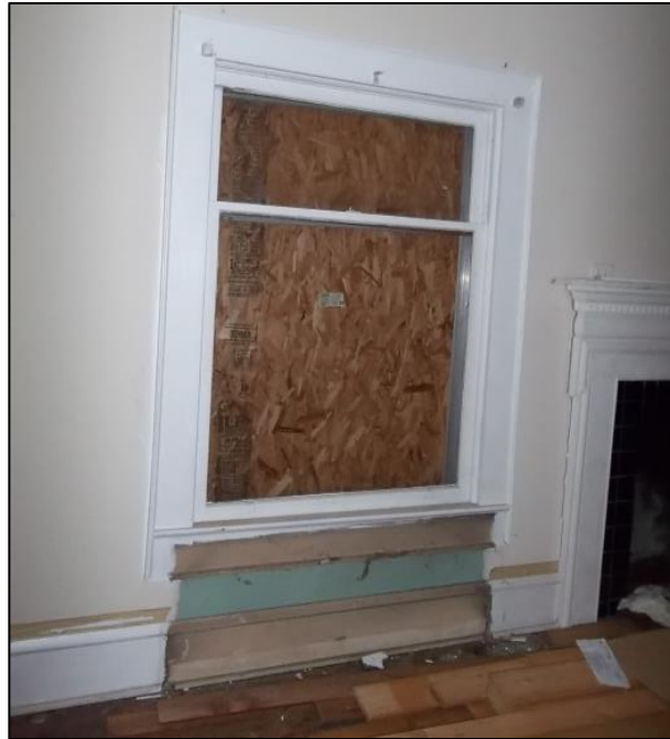
Photo 44: Replacement First Story Window Looking West From Inside the House.
