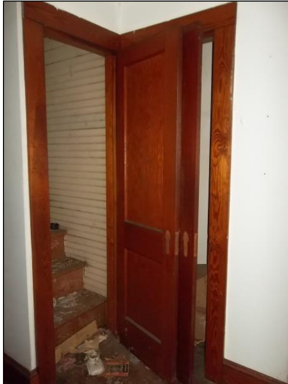
Photo 69: Attic Stairwell, Looking Northeast.
