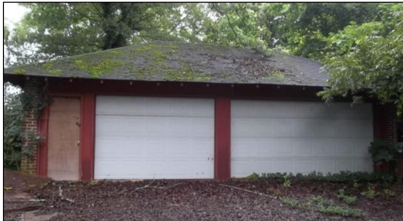
Photo 29: East Elevation of the Garage.
