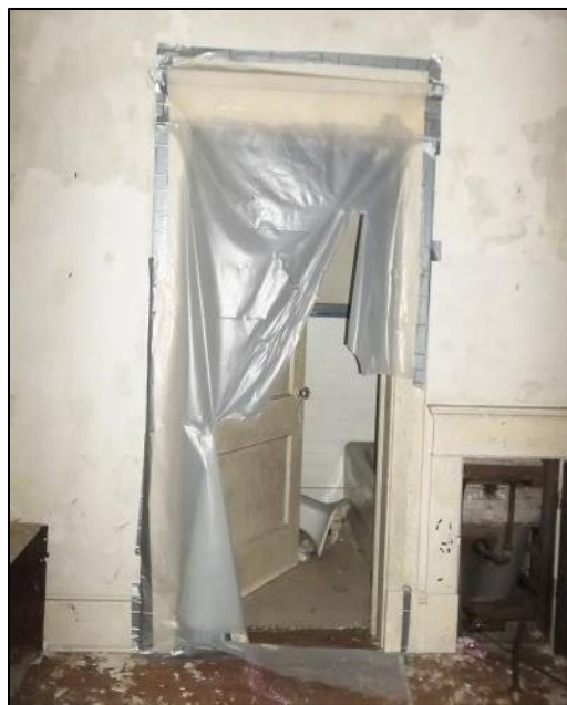
Photo 17: View into the First Story Bathroom, Looking West.
