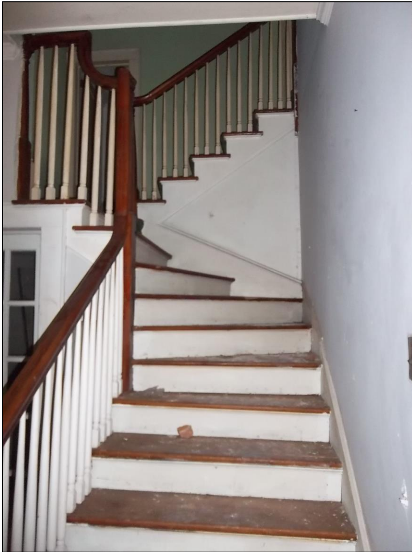
Photo 57: Main Staircase, Looking East.
