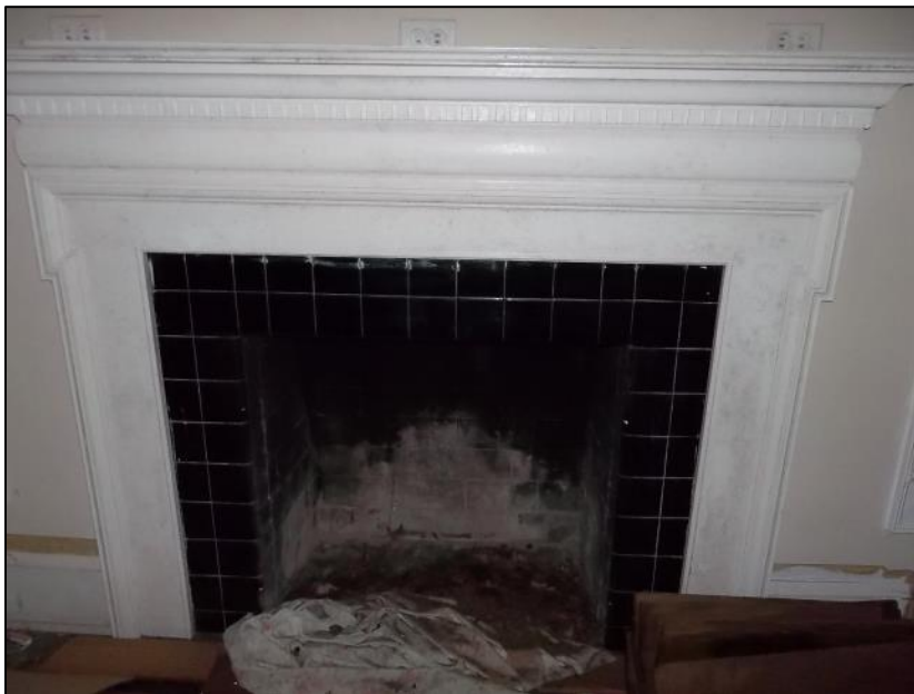
Photo 59: Detail of Fireplace in the Southwest Room.
