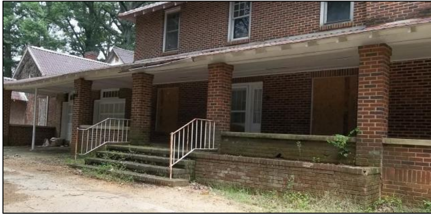
Photo 46: Detail of the Porch, Looking Northeast.
