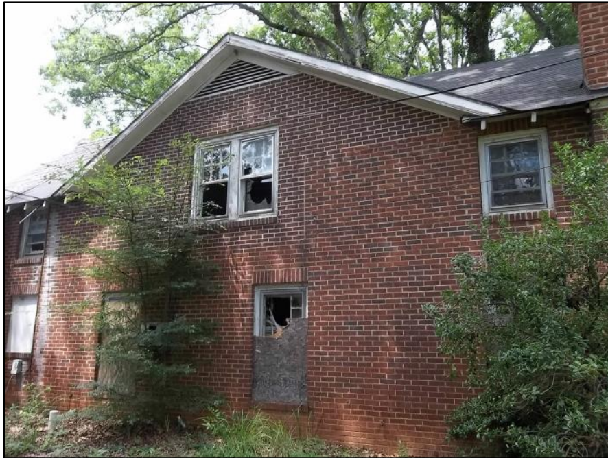
Photo 51: South Elevation of the Apartment Addition.
