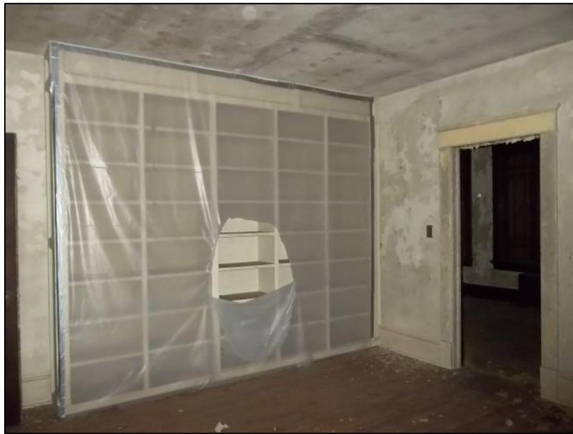
Photo 16: Library, Looking Northeast.
