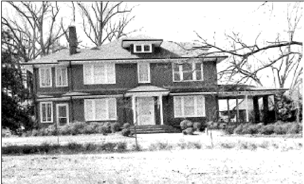
Photo 1: 1980 Photograph of the East Elevation of the R.O. Caldwell House (North Carolina Department of Cultural Resource Resources 2013).
