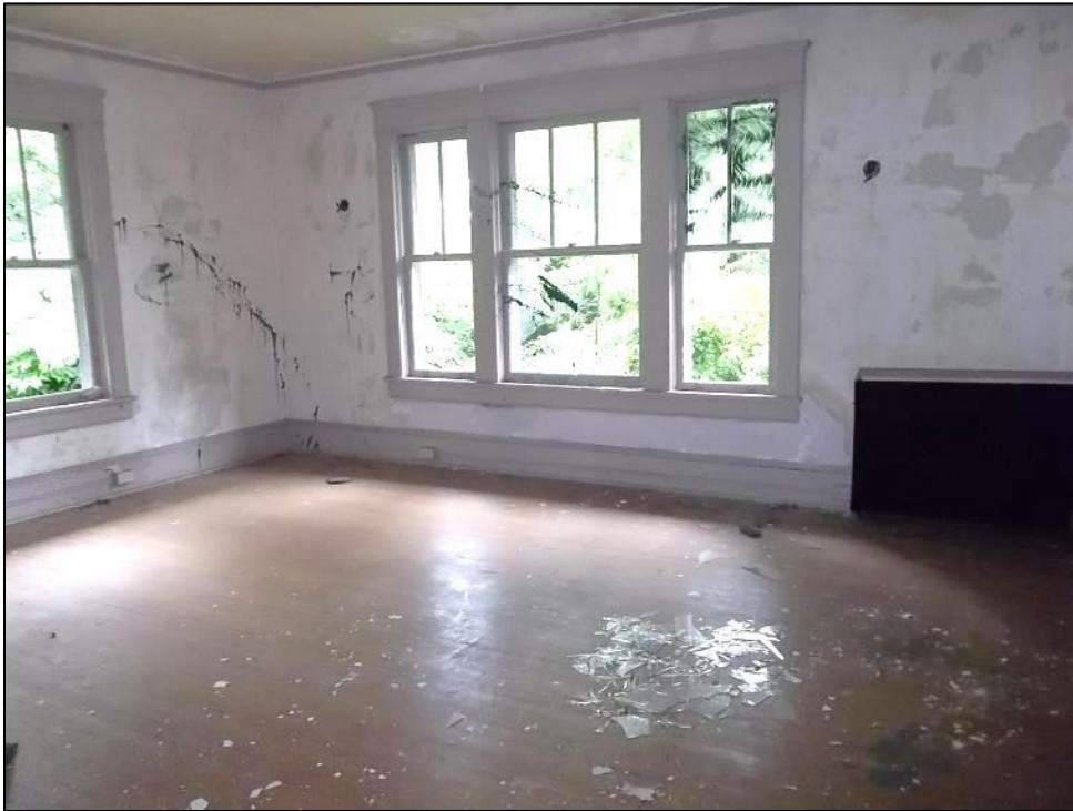
Photo 23: Bedroom at the Southeast Corner of the House, Looking Southeast.
