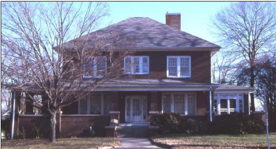
Photo 39: Primary Elevation of the Circa-1923 Harvey Jeremiah Peeler House (CA 1072), Kannapolis, North Carolina (Cabarrus County Information Technology Services 2013).
