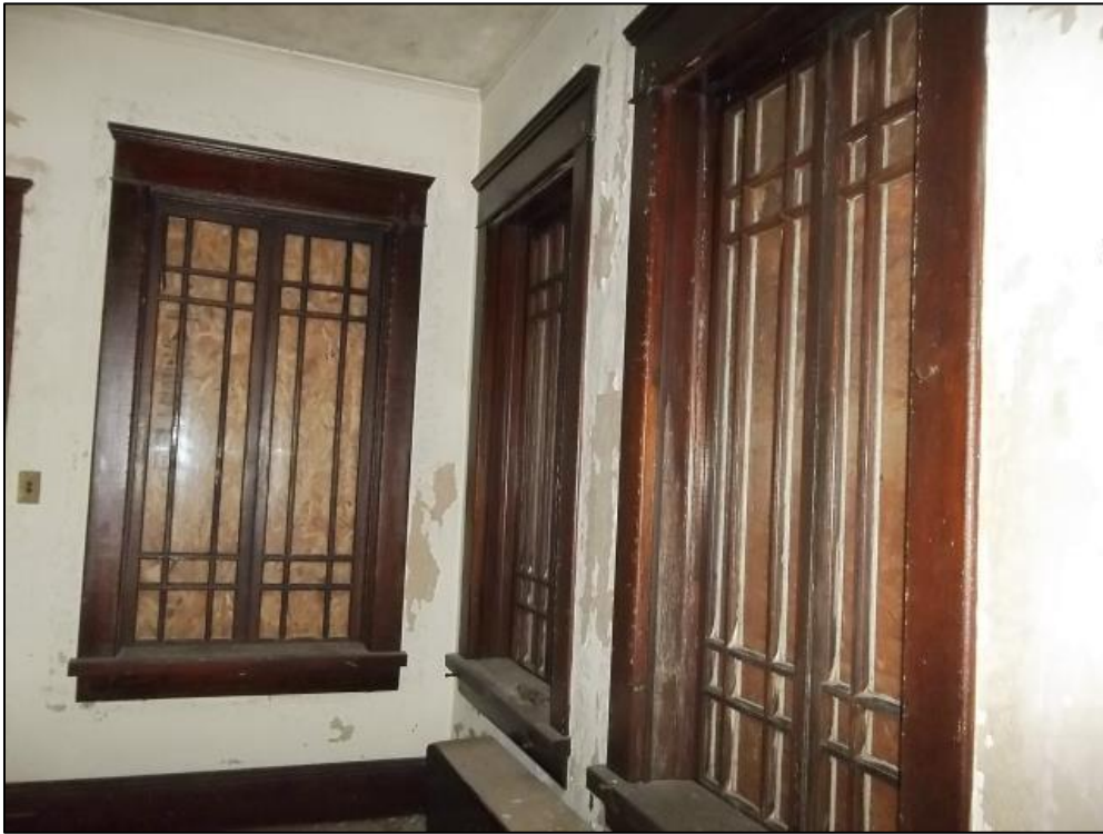
Photo 21: First Story Sunroom, Looking at Southwest Corner.
