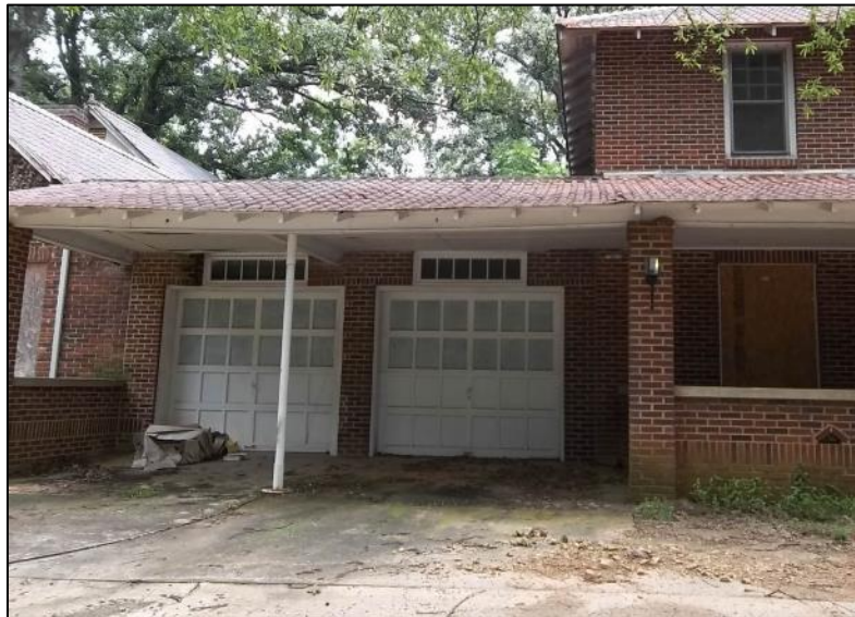
Photo 54: West Elevation of the Garage.
