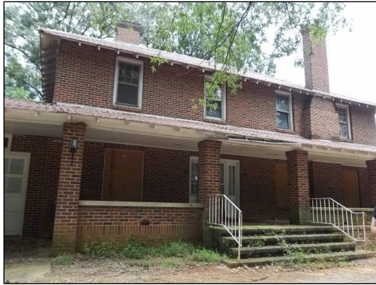
Photo 42: West Elevation of the Dr. H.W. Barrier House.
