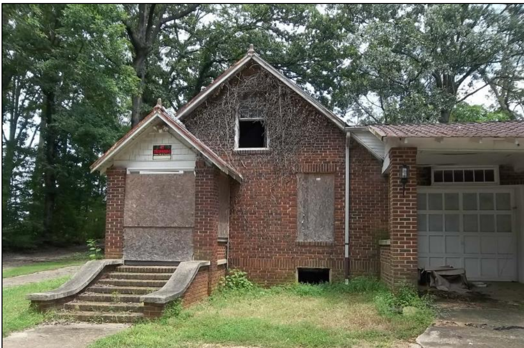
Photo 48: West Elevation of Dr. Barrier's Office.
