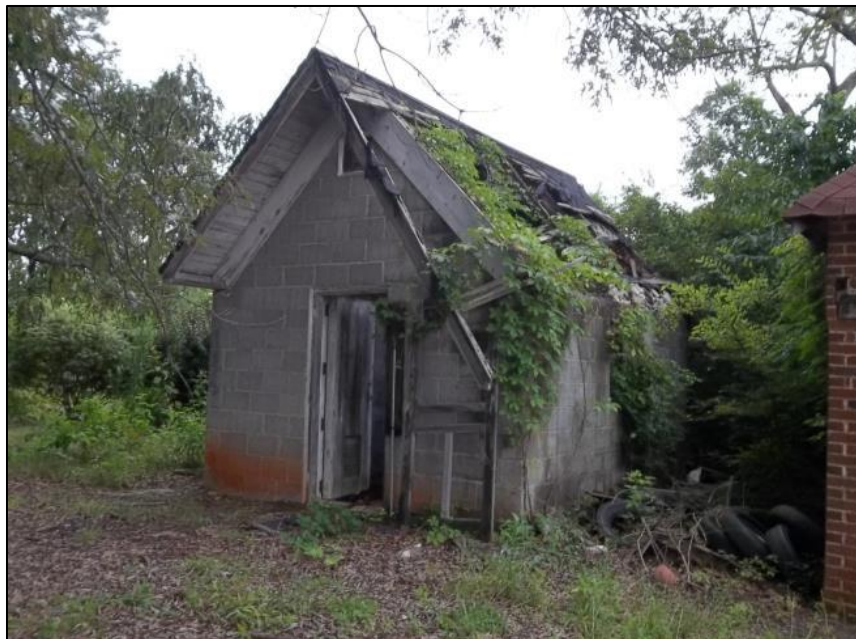
Photo 79: Southwest Oblique of the Shed.
