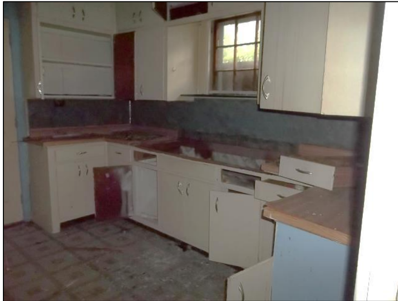
Photo 78: Apartment Kitchen Overview.
