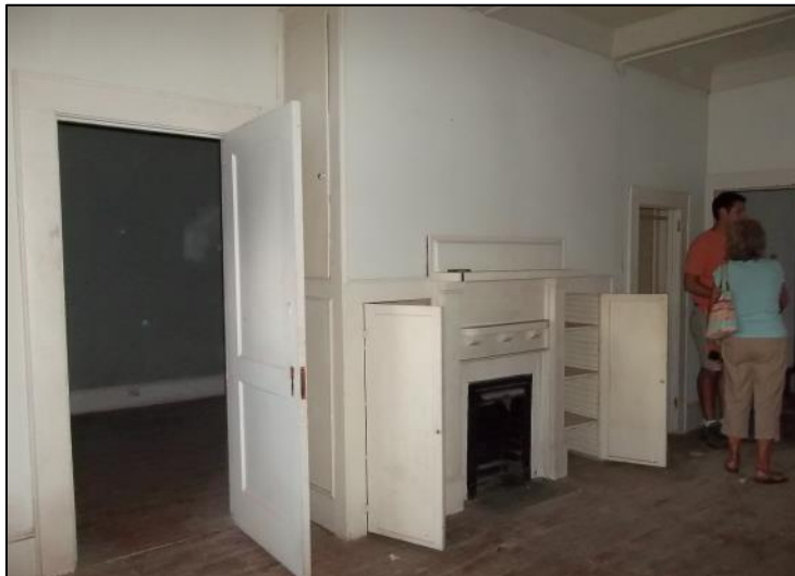
Photo 61: Southeast Room Looking Northwest Toward the Fireplace.
