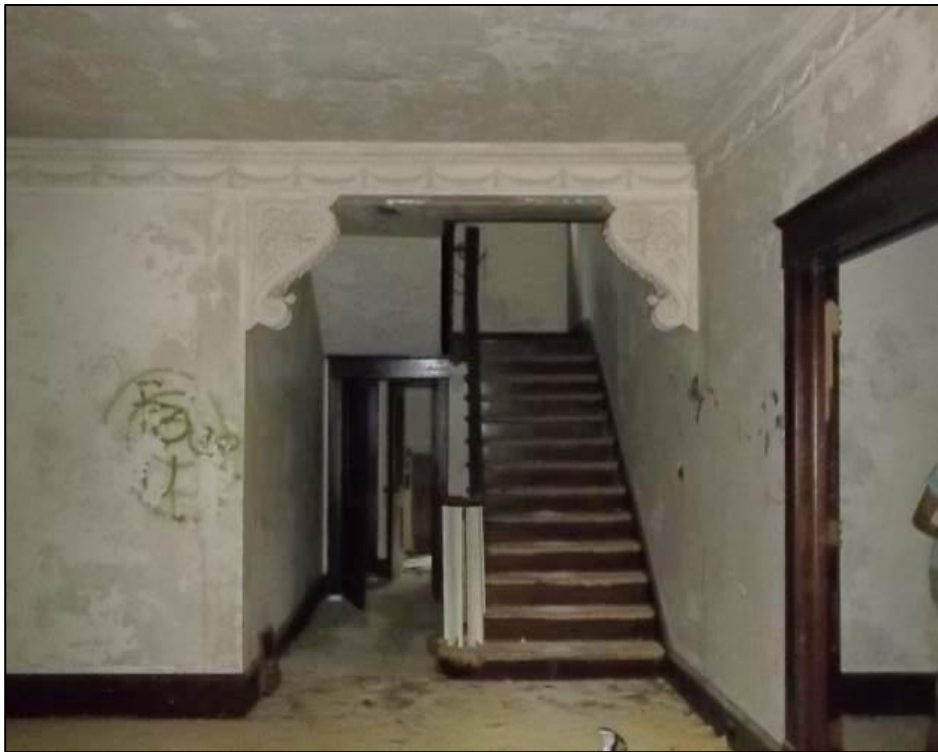
Photo 15: View of the Staircase, Baseboards, Brackets, and Crown Molding, Looking West.
