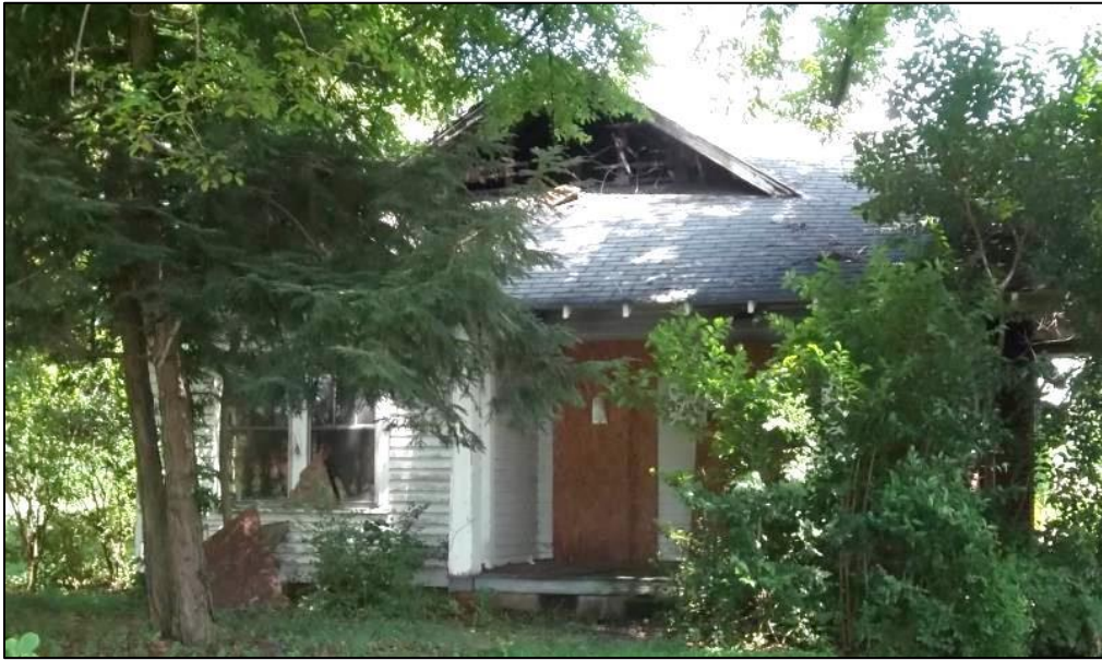
Photo 32: South Elevation of the Secondary Dwelling.
