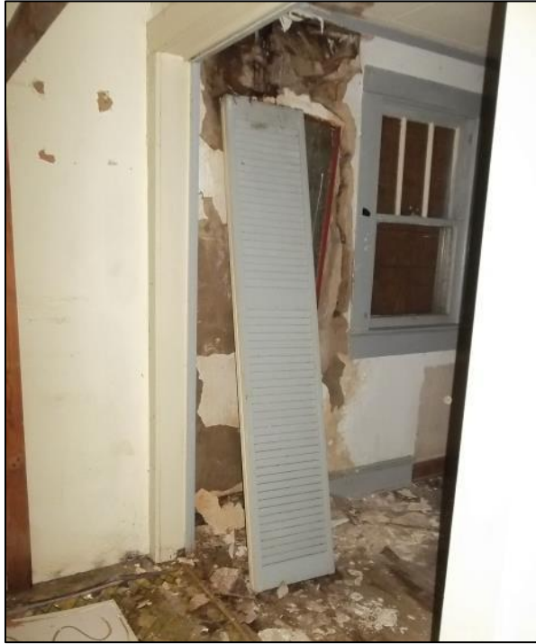
Photo 68: Bedroom on the Second Floor, Looking Southeast.
