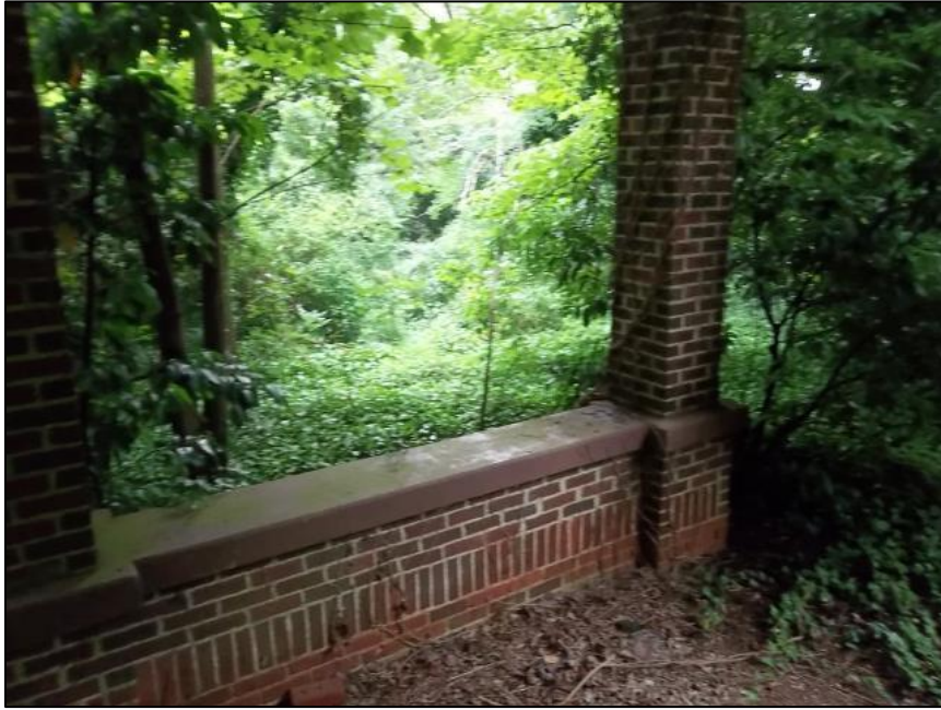
Photo 6: Porte-Cochère Wall, Looking Northeast.
