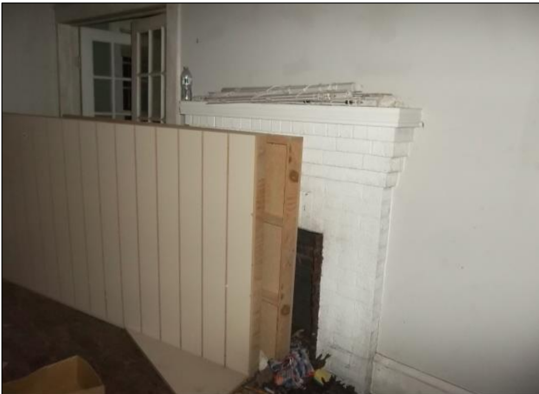
Photo 56: Detail of the Brick Fireplace in the Northwest Room, Looking Northeast.
