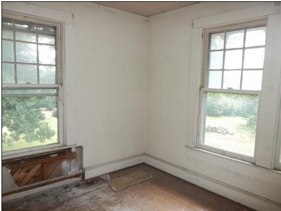
Photo 67: Southeastern-Most Bedroom on the Second Story.
