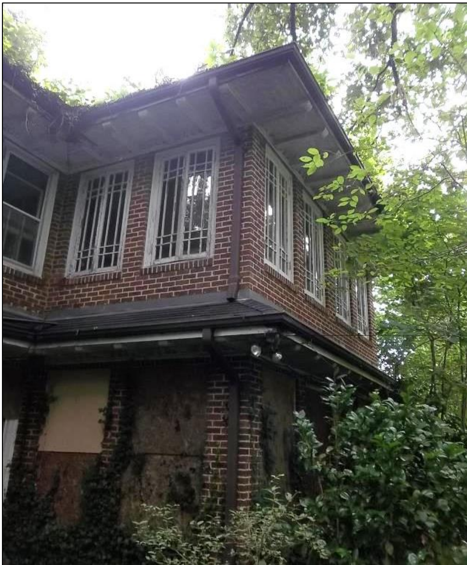
Photo 10: Southwest Elevation of the Two-Story Sunroom.
