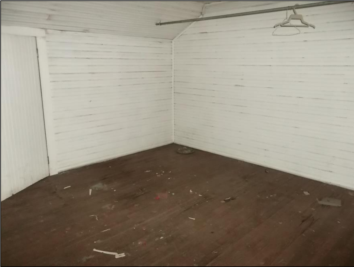
Photo 25: Attic, Looking Southeast.
