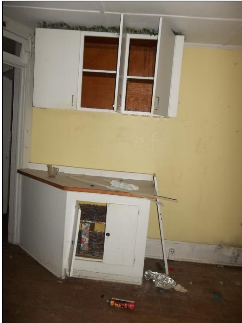
Photo 75: Southeastern Office Remodeled to be a Kitchen.
