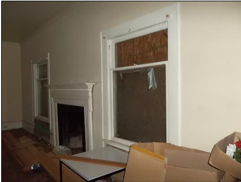
Photo 58: Southwest Room, Looking Southwest Toward the Fireplace.
