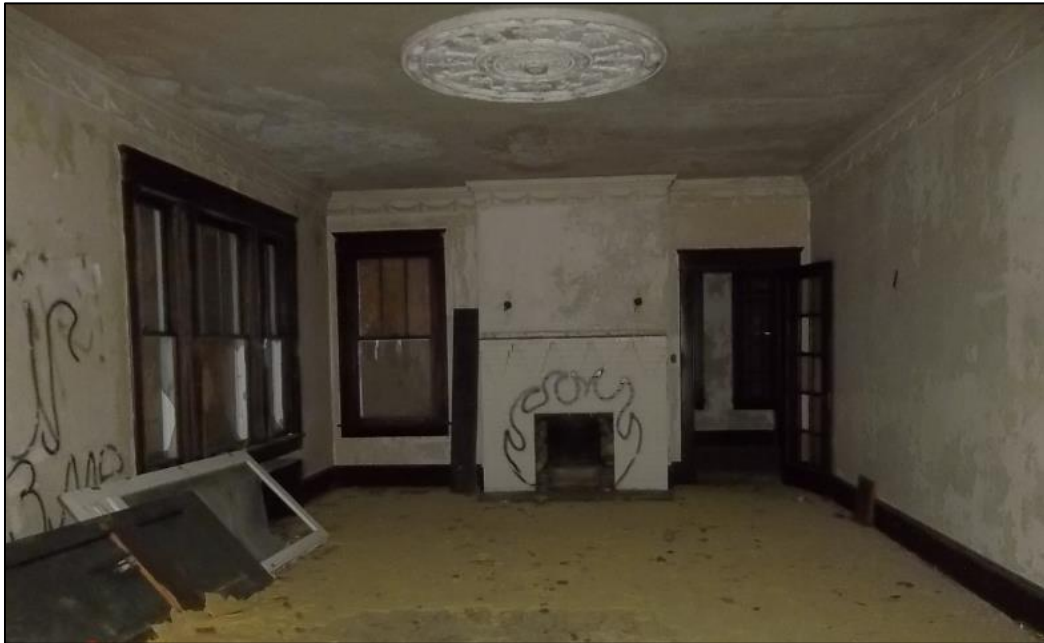
Photo 12: Overview of the Main Room on the First Story, Looking South.
