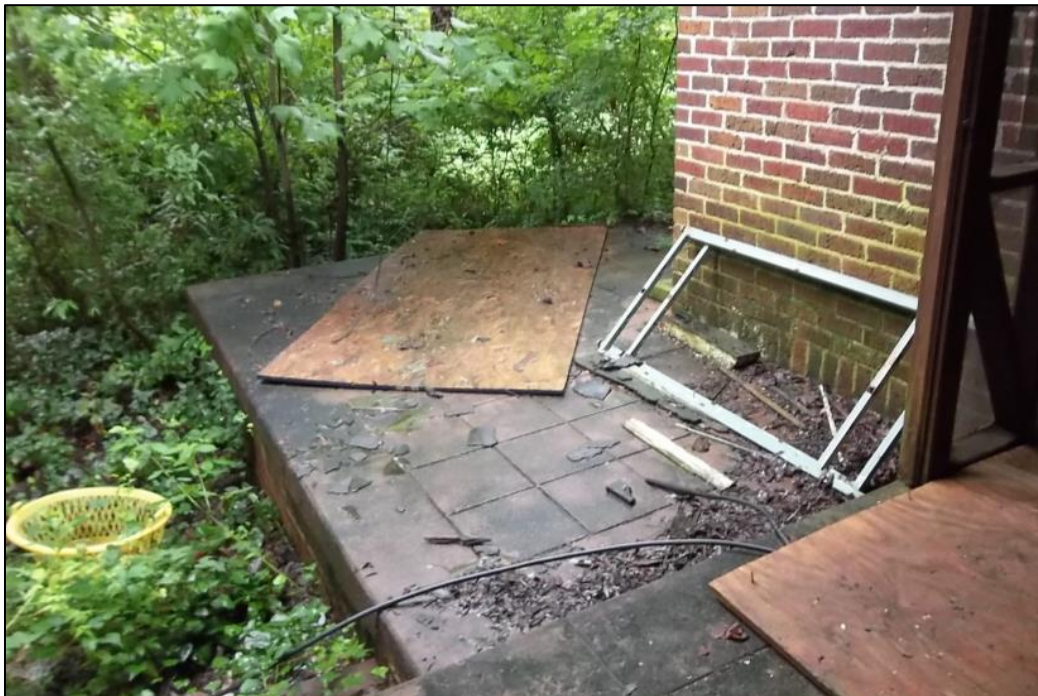
Photo 5: Detail of the Walkway that Connects the Front and Side Porches.
