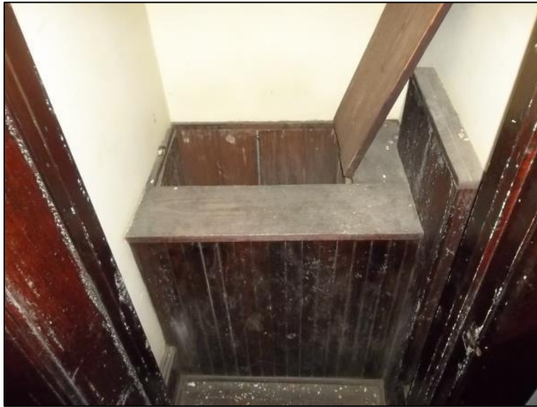
Photo 18: First Story Laundry Chute.
