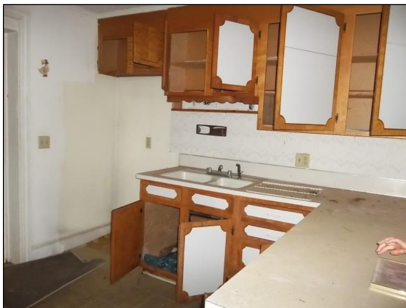
Photo 71: Kitchen Located on the Second Story, Looking Southwest.
