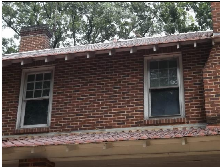
Photo 45: Detail of the Second Story Windows.
