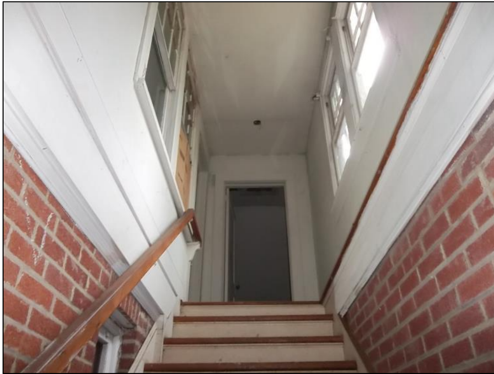
Photo 76: Looking South in the Apartment Foyer Addition. The original exterior wall of the apartment is on the left and the current foyer exterior wall is on the right
