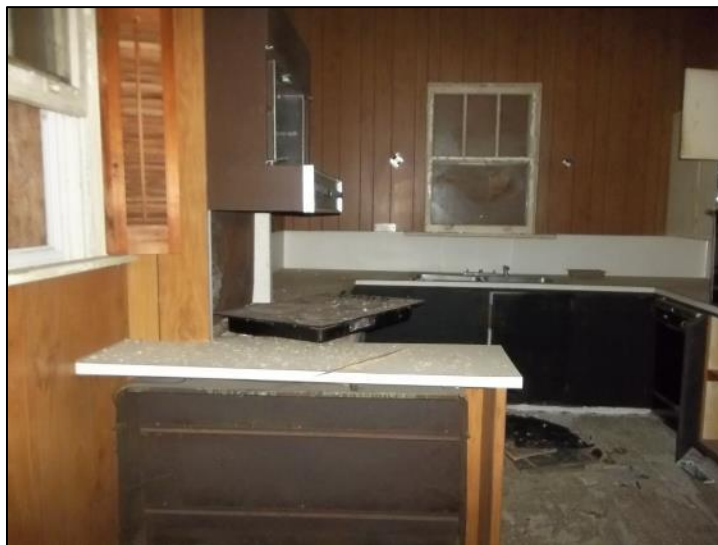
Photo 19: Kitchen, Looking North.
