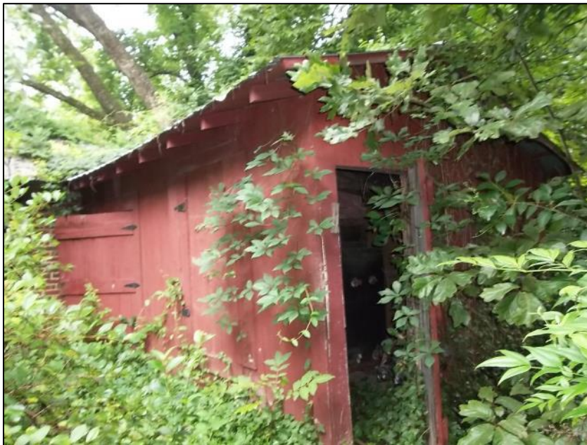
Photo 27: One-story, Frame Shed Attached to Smokehouse, Southeast Oblique.
