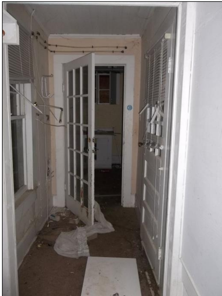
Photo 72: Walkway from Main House to Office, Looking North Toward the Office.
